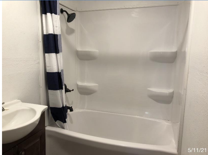
New tub and shower insert, refinished walls and floor in the main bath.
