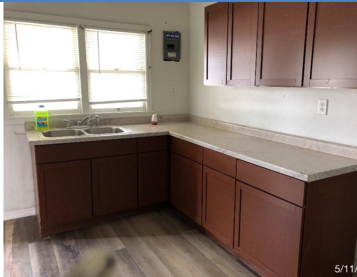
Refinished kitchen including new cabinets, countertop, and laminate floor.
